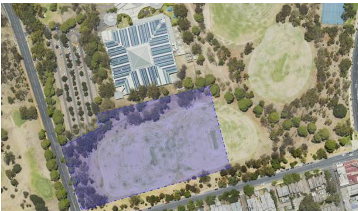
Image 2 – Temporary Works Compound (Stage 1 – 25,000 sqm)
