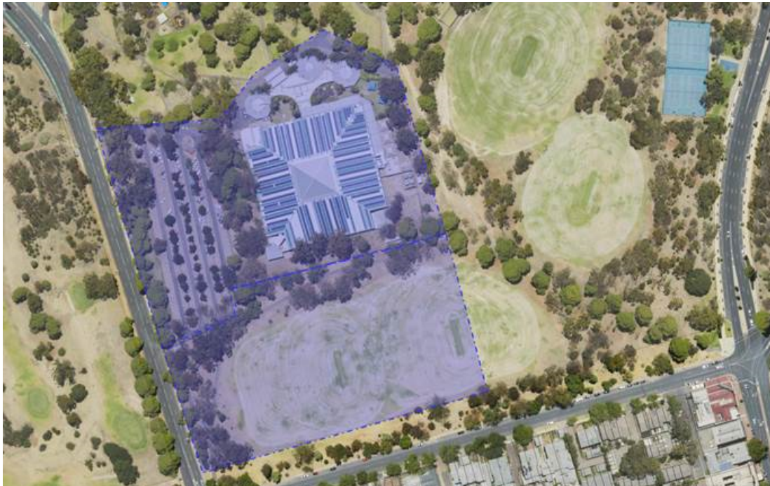
Image 3 – Temporary Works Compound: (Stage 2 – 35,000 sqm)
